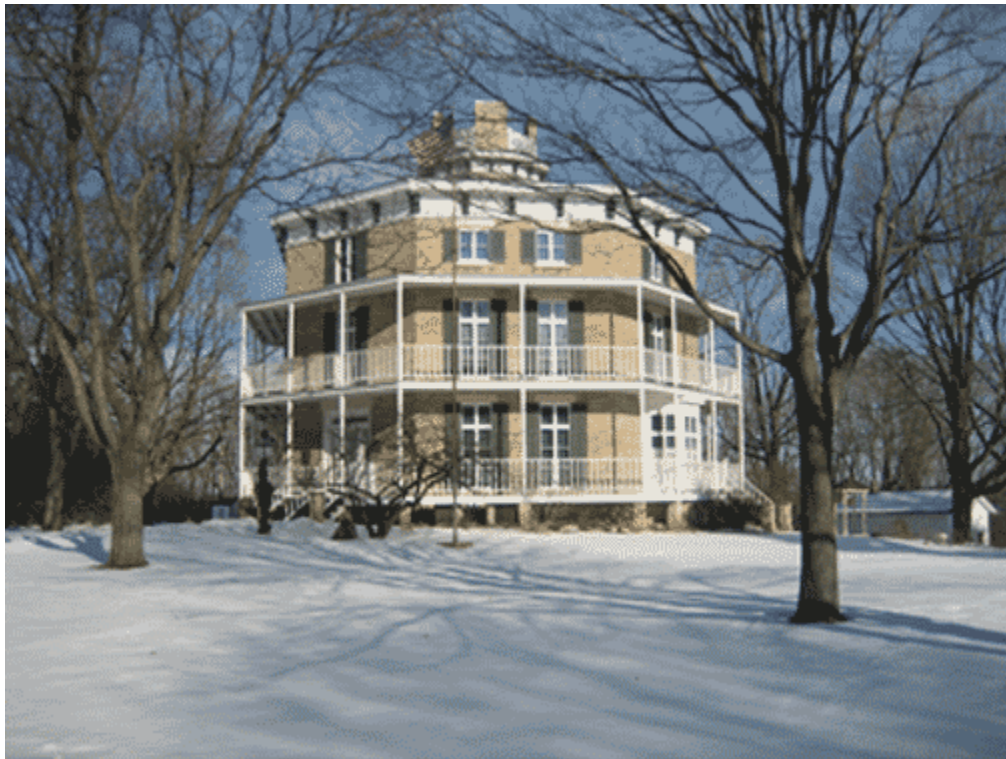
Richards octagon house, Watertown, Wisconsin, completed in 1854.
